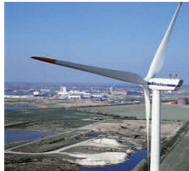
(Left) Despite its length, the LM 61.5P blade weighs only 17,740 kg/39,110 lbs. (Photo courtesy of LM Glasfiber)
